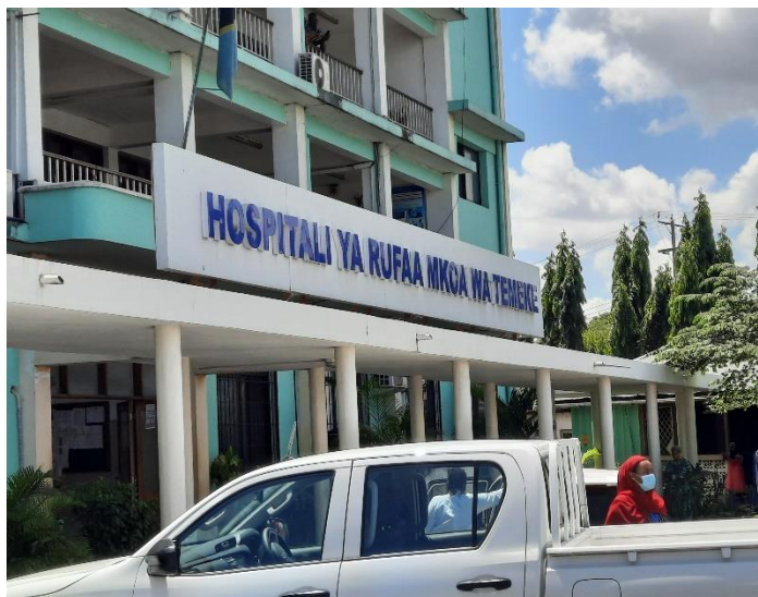
Front view of Kemeke Regional Hospital
