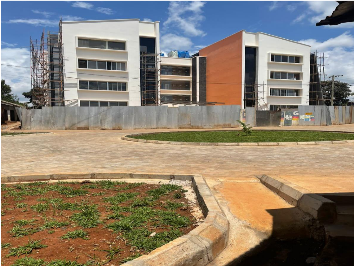
Ultra-modern integrated laboratory complex under construction at KIDH
